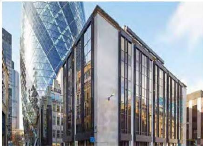
View from Creechurch lane
